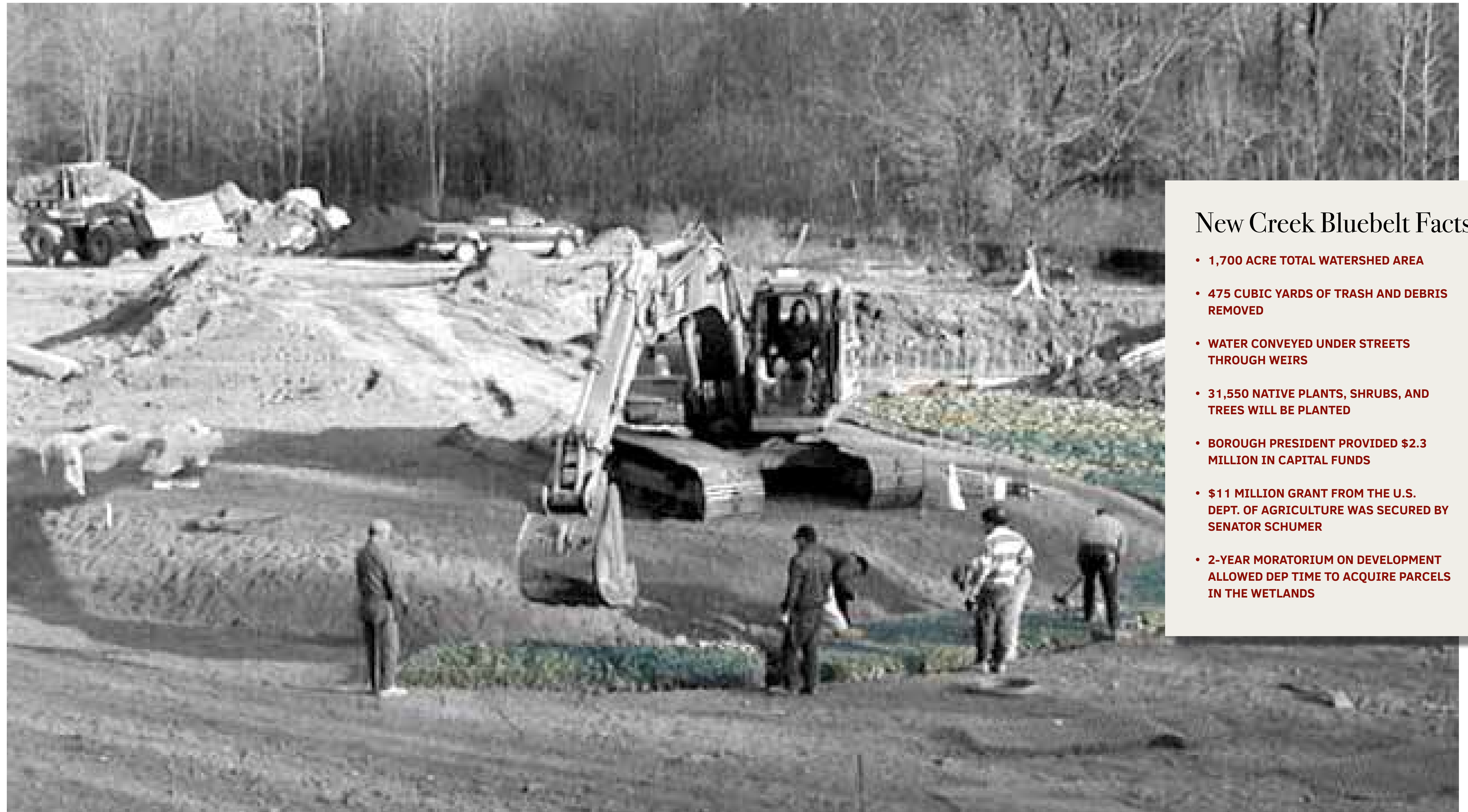
DEP engineers deepen natural stream corridors to create functional Bluebelt flood protection for neighborhoods.
